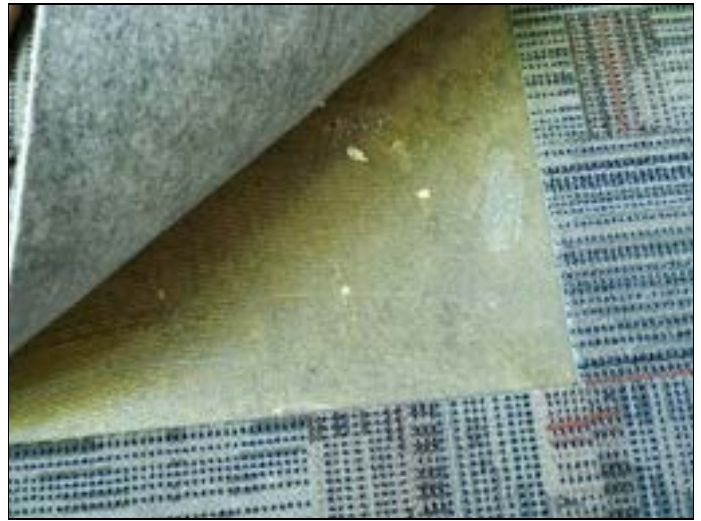
26. Samples 20A-20C: Yellow carpet mastic, first floor
