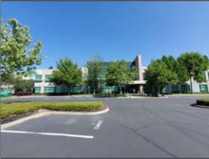
1. 11931 Foundation Place, overview of property exterior
