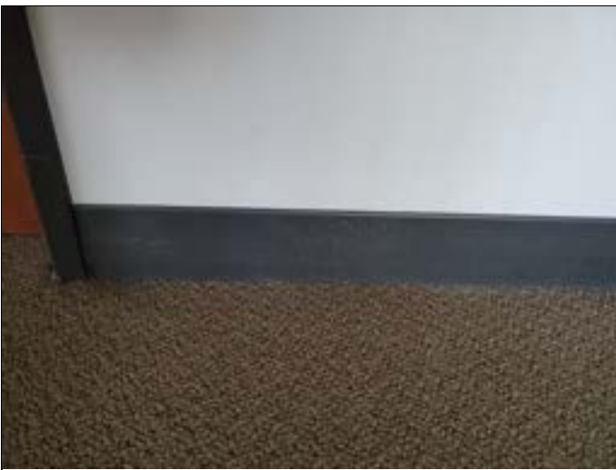
11. Samples 05A-05C: 4" brown cove base with cream mastic, second floor
