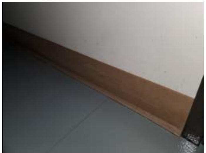
18. Samples 12A-12C: 4" yellow-brown cove base with tan mastic, second floor
