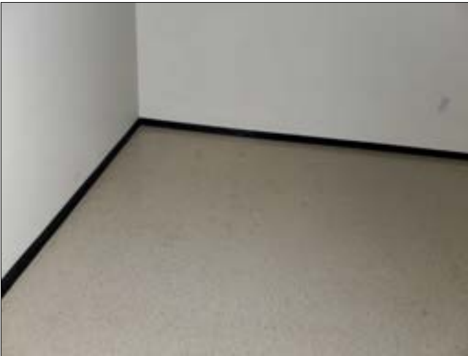
21. Samples 15A-15C: 3" black cove base with light brown mastic, first floor
