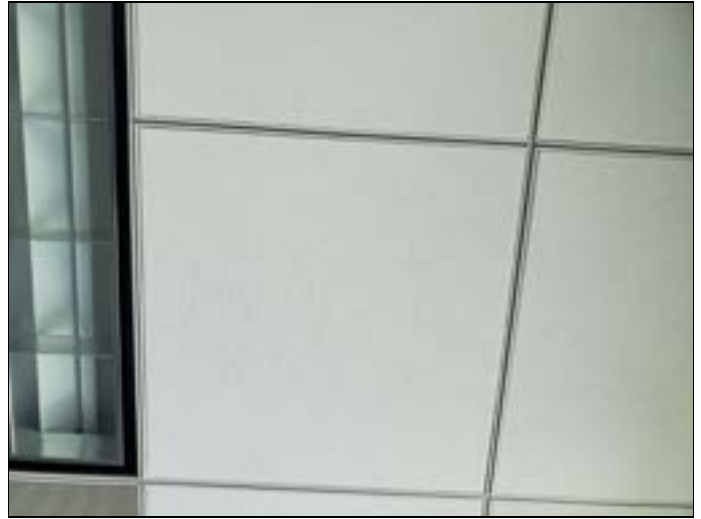
20. Samples 14A-14C: 2'x2' ceiling tile with rough texture, first floor
