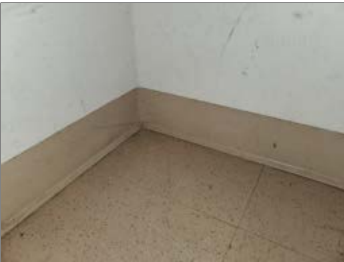
9. Samples 03A-03C: 4" beige cove base with tan mastic, second floor
