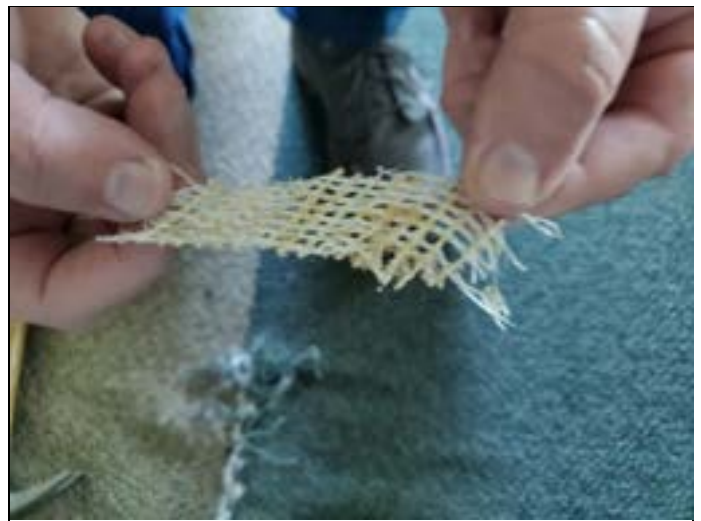
12. Samples 06A-06C: Yellow carpet mastic with white leveling compound, second floor
