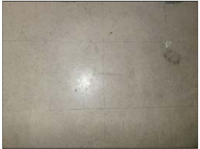
8. Samples 02A-02C: 12"x12" beige VFT with black specks and yellow mastic, second floor
