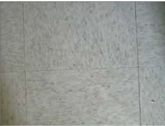
17. Samples 11A-11C: 12"x12" grey mottled VFT with yellow mastic, second floor
