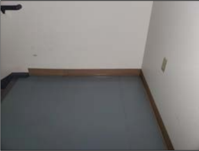
19. Samples 13A-13C: Grey plain VSF with white mastic, second floor
