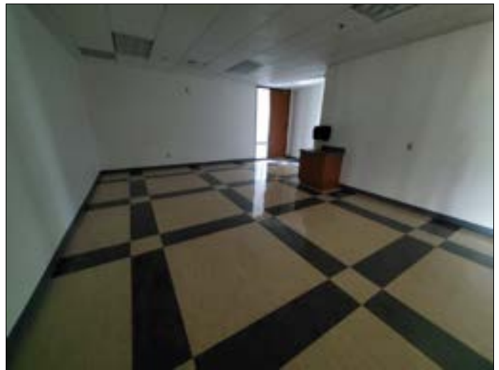
16. Samples 10A-10C: 12"x12" grey and beige patterned VFT with yellow mastic, second floor
