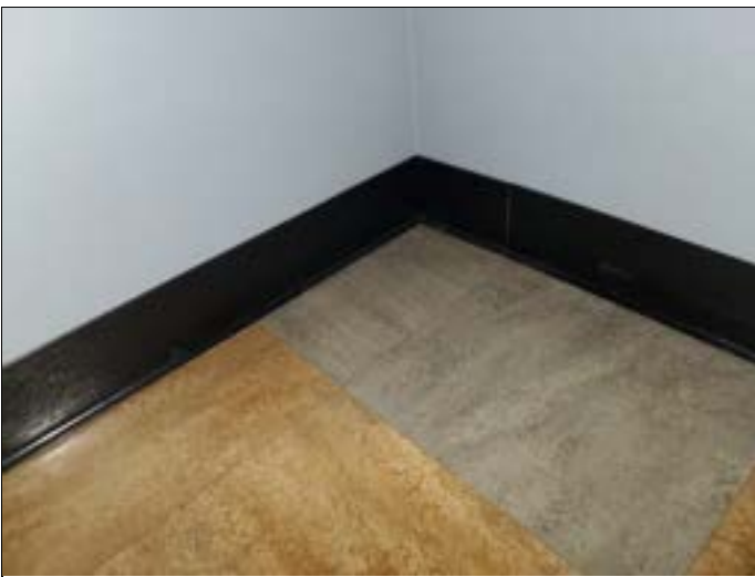
29. Samples 23A-23C: 4" black cove base with white mastic, first floor
