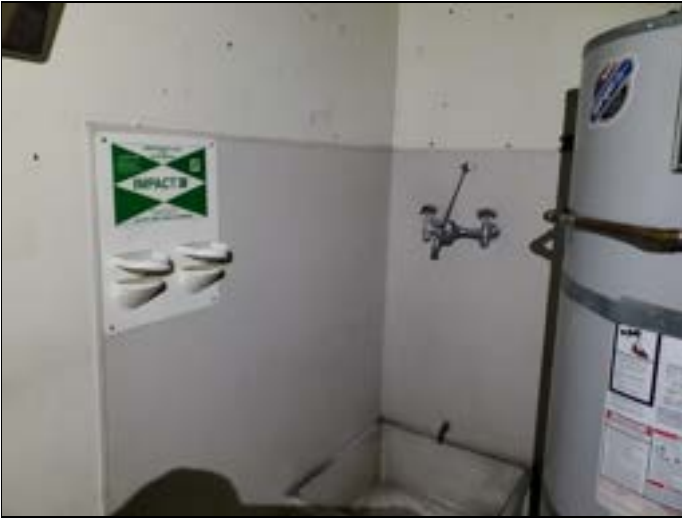
37. Assumed ACM: Mastic associated with fiberglass panels, second floor roof access room
