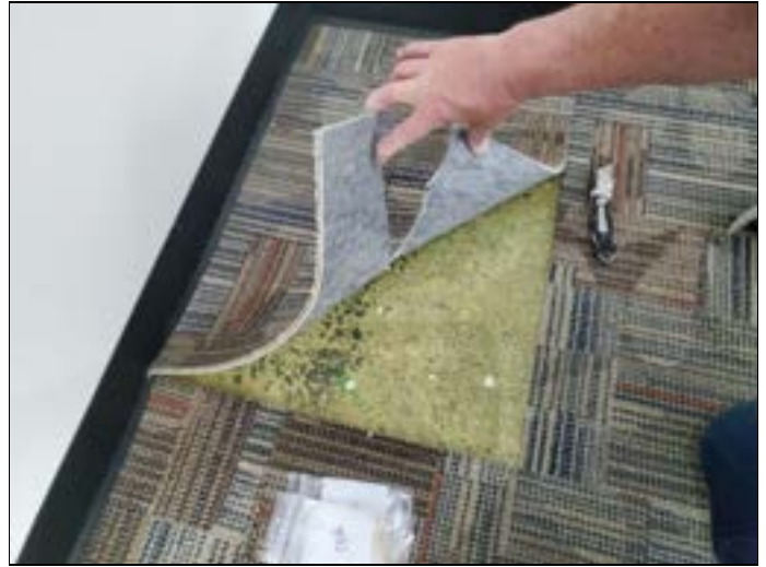
14. Samples 08A-08C: Yellow and blue carpet mastic, second floor
